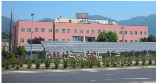
ASM Terni buildings + 60 kW PV
